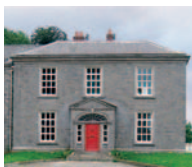
Above The mill house
